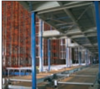
Mezzanine construction at the infeed - outfeed of the AS/RS-system
